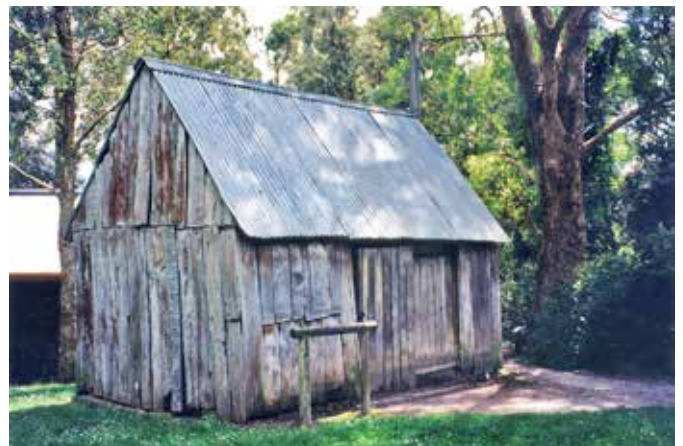
The Blacksmith’s shop or ‘Smithy’ was erected from timbers found in a paddock in the Dandenong Ranges by Mr George Cox, which were transported to the Cottage site and re-erected in 1970 on a part of the site where remains of a previous building had been found.
